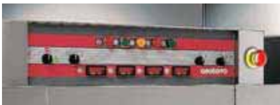
Electrical panel with protected control devices supplied at low voltage.
